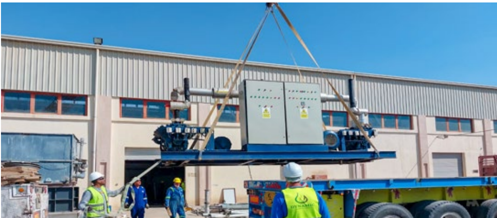
Re-allocating Ammonia chillers with installations and commissioning
