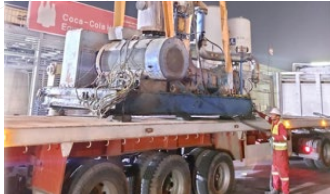
Relocating and installing high pressure compressor AF with commissioning
