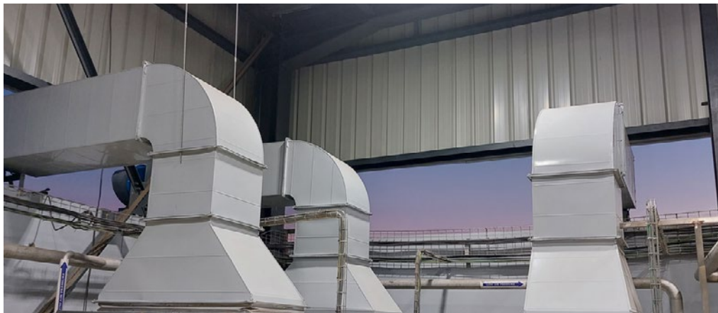
Installing a compressed air system with an exhaust duct
