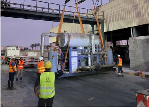
Supplying and fabricating new syrup dissolving unit
