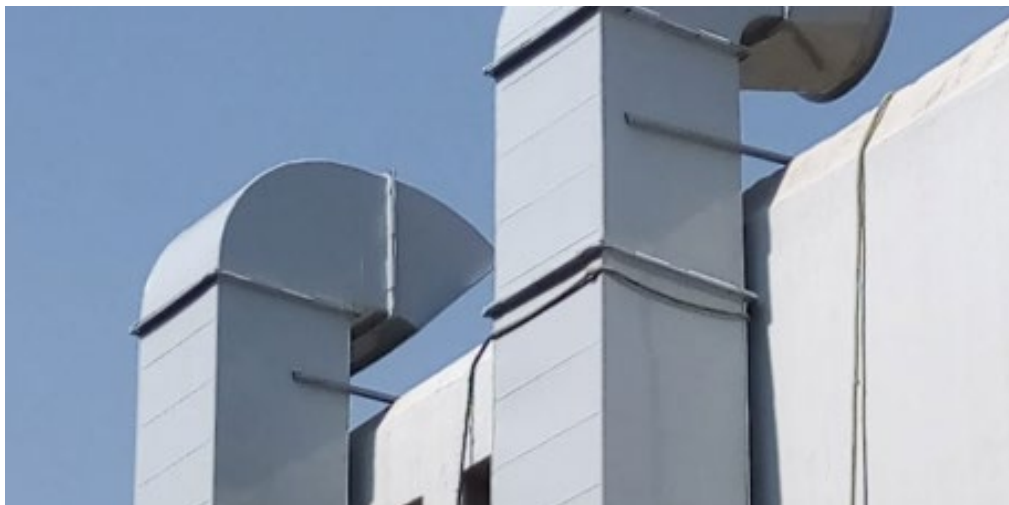
Installing a compressed air system with an exhaust duct
